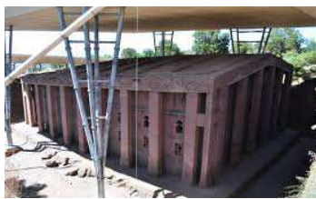
Figure 4.4 the New Shelter Constructed by UNESCO and European Union
