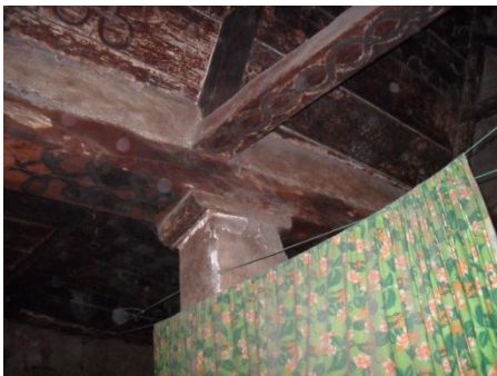
Figure 3. 21: Capitals supporting arches in the church of Yimrehane Kiristos (above) and lintels rested on wooden capitals in the church of Imekina Medihanialem (below)
