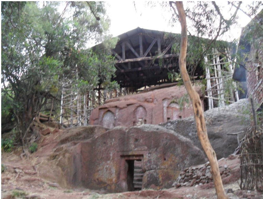
Figure 3. 13: Semi-monolithic church of Bilbala Kirkos; a framed (formed in recess) entrance to the courtyard, western facade of the church with blind arches and shelter
