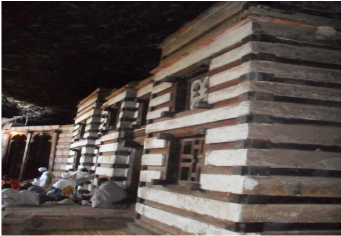
Figure 3. 17: Cave Church of Yimrehane Kiristos; northern facade
