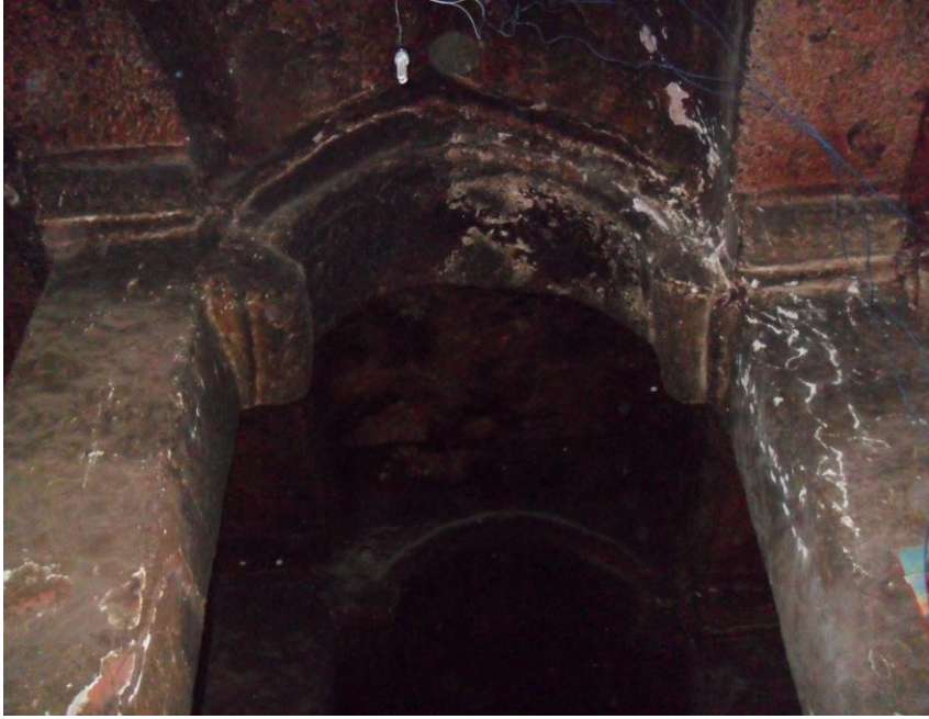
Figure 3. 12: Eastward view from central nave area into the sanctuary; arches, lintels, columns with roughly worked bracket capitals
