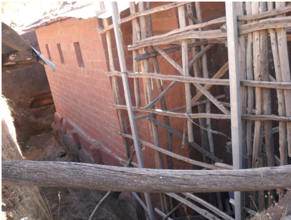
Figure 3. 16: renewed part of the church, eastern facade
