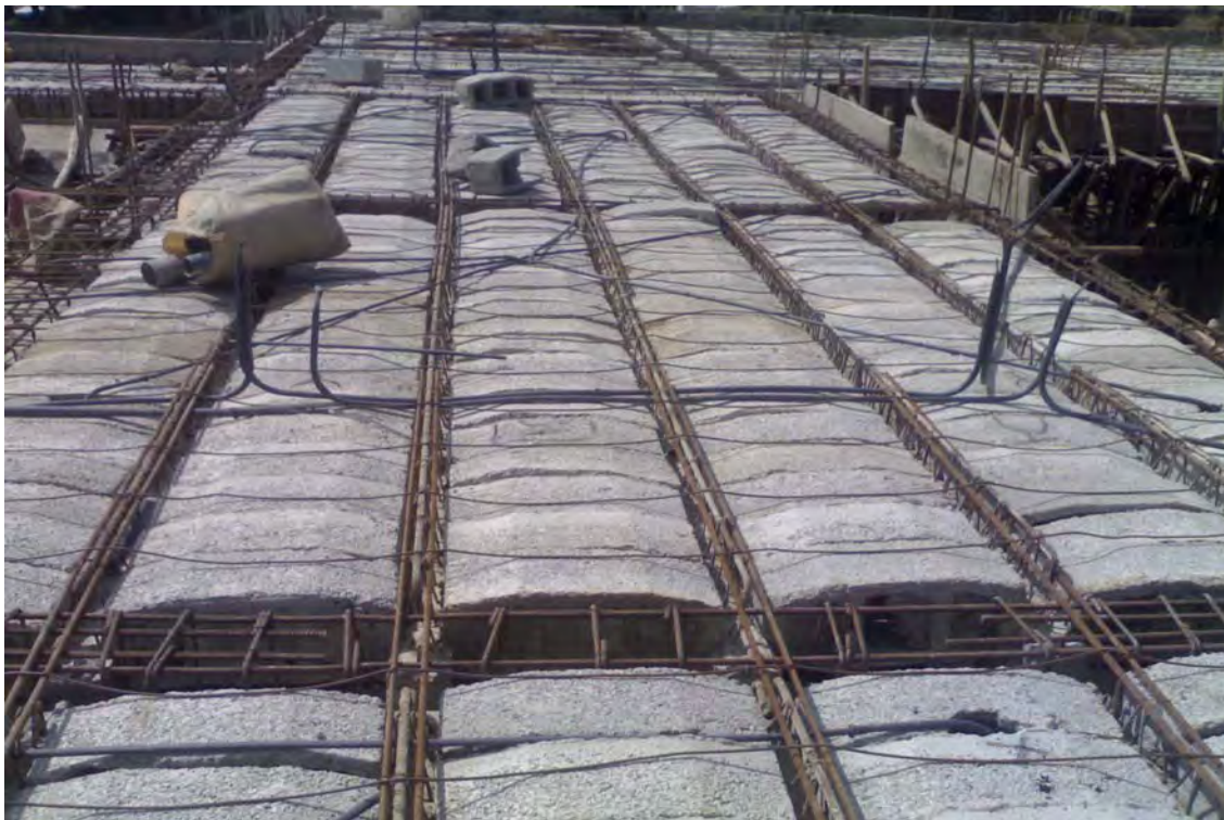
Fig1.10 Pre-cast Beam-Slab prior to concreting.
