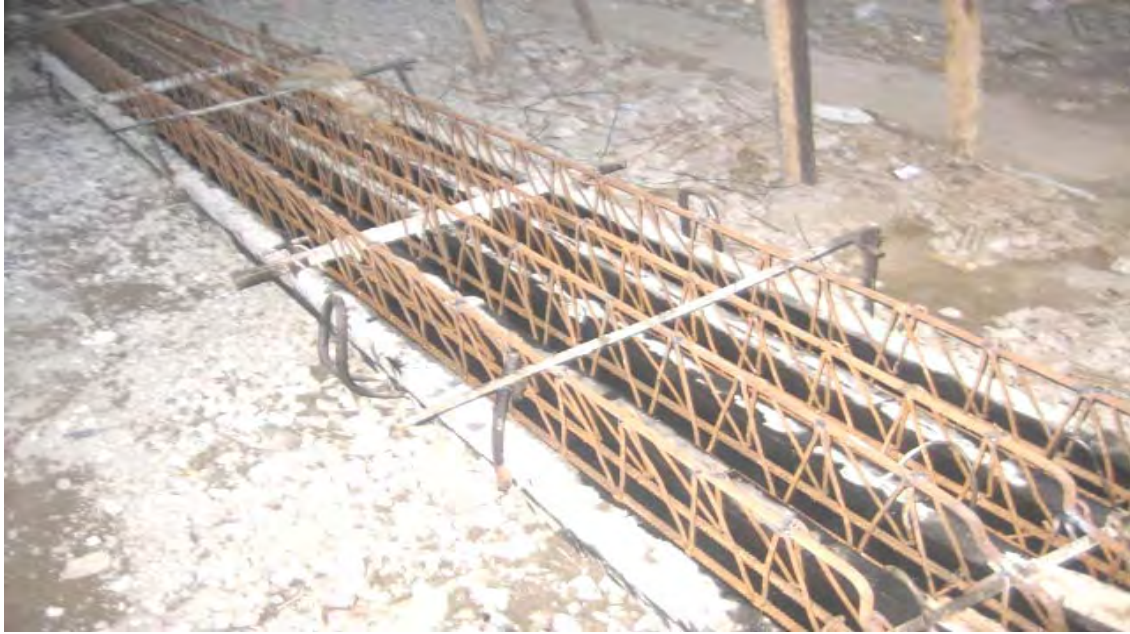
Fig. 2.6 Reinforcements welded and put in the mould.
