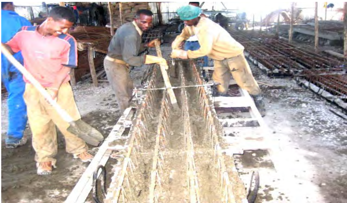
Fig. 2.7 Concrete Placing.
