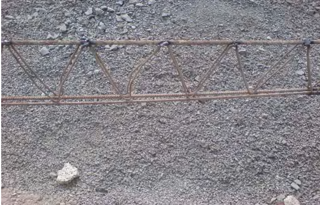
Fig1.9 Reinforcement welded at all nodes.
