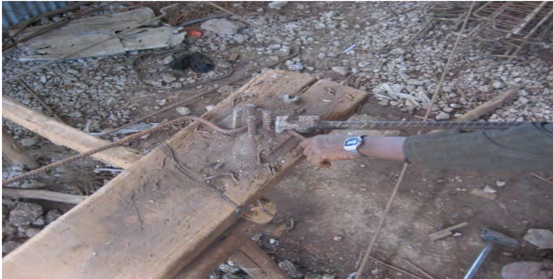
Fig.2.4 Bending of the main reinforcement.
